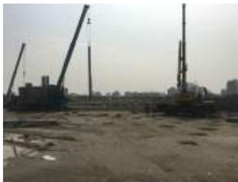
Pre Cast Pile Pictures
