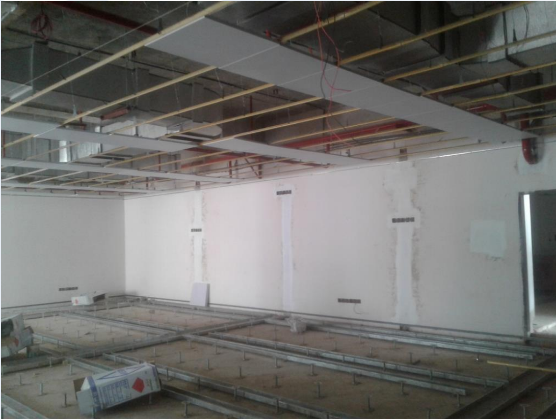
Elevated Floor & False Ceiling Work
