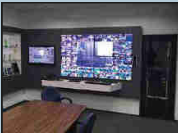
Wasa Control Room Design
