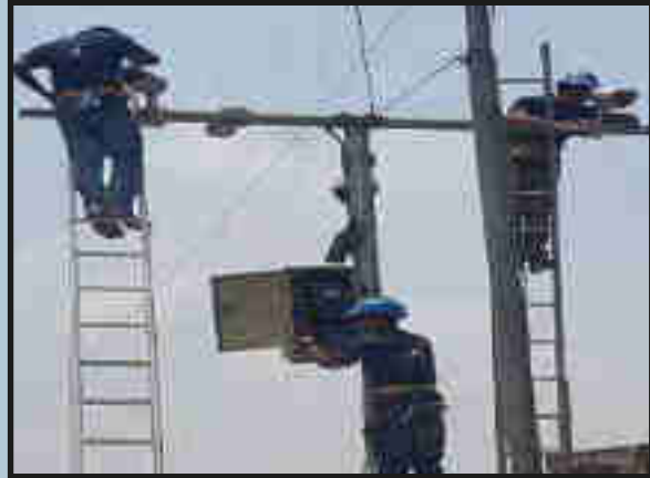
Meghna group of industries Economic Zone Project
