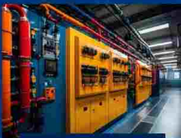
Power Generator (Genset)
